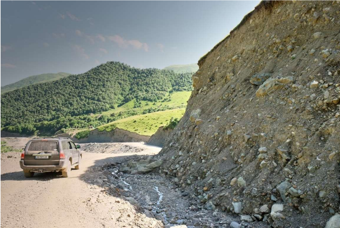
Picture 2: Newly upgraded road to Roshka National Monument – detail of the exposed slope inviting further erosion.
