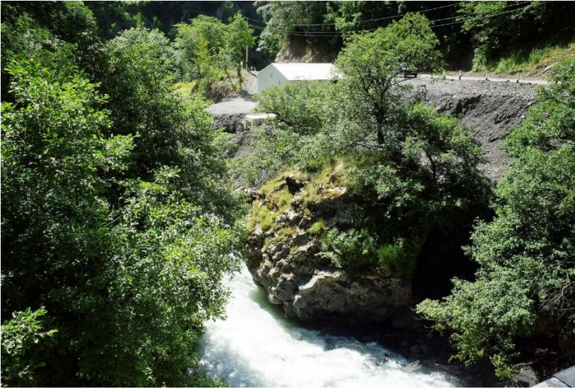
Picture 3: A new small HPP under Roshka
