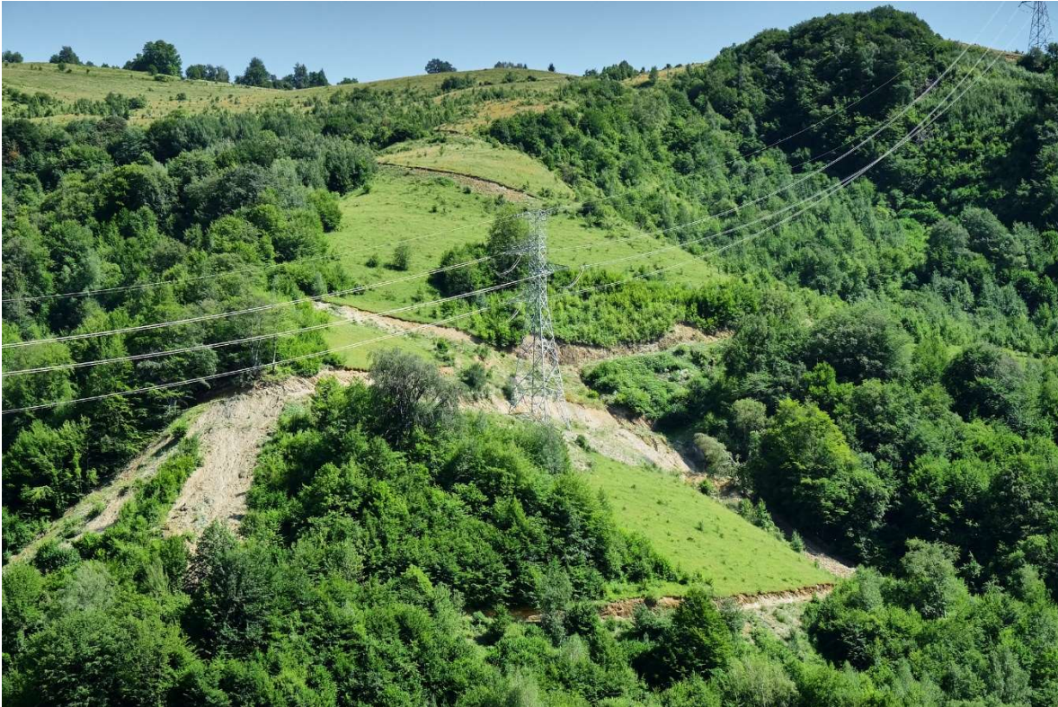
Picture 1: A newly built power line post near Kitokhi village
